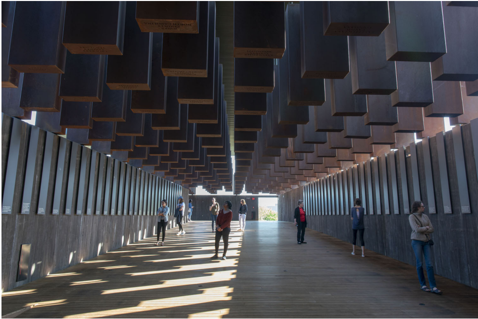
Figure 8. National Memorial for Peace and Justice, Montgomery, Alabama, 2018. Photograph by Alan Ricks, provided by MASS Design Group.
